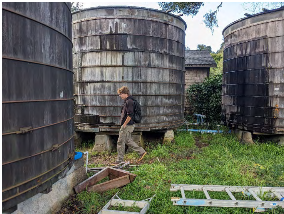
Photo 1. Location of the three water tanks to be replaced.
